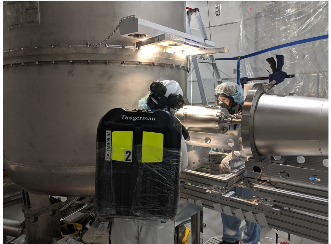
Derek Lucero (front) and I sealing the inner cone to the ICV. Oxygen masks had to be worn because of the N_2 purge.
