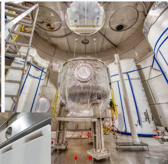
OD tanks and OCV in the water tank
